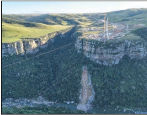
Left: The bridge is being built from the north and south banks of the gorge and comprises two identical 'halves', each spanning 290 m, which will meet mid-point over the gorge.
