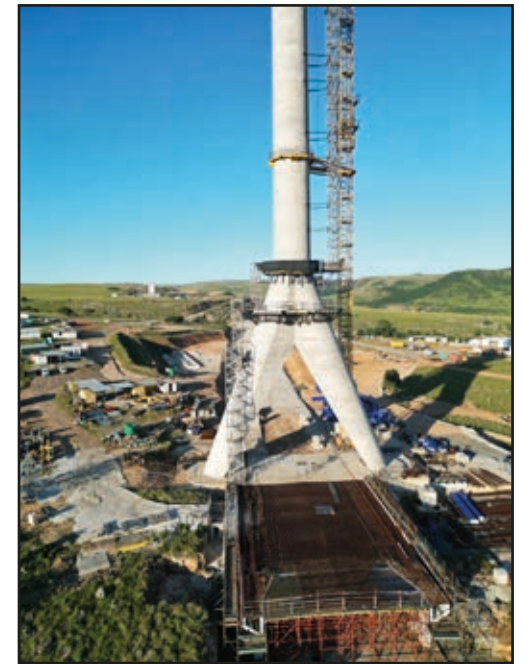
Left: The bridge is being built from the north and south banks of the gorge and comprises two identical 'halves', each spanning 290 m, which will meet mid-point over the gorge.
