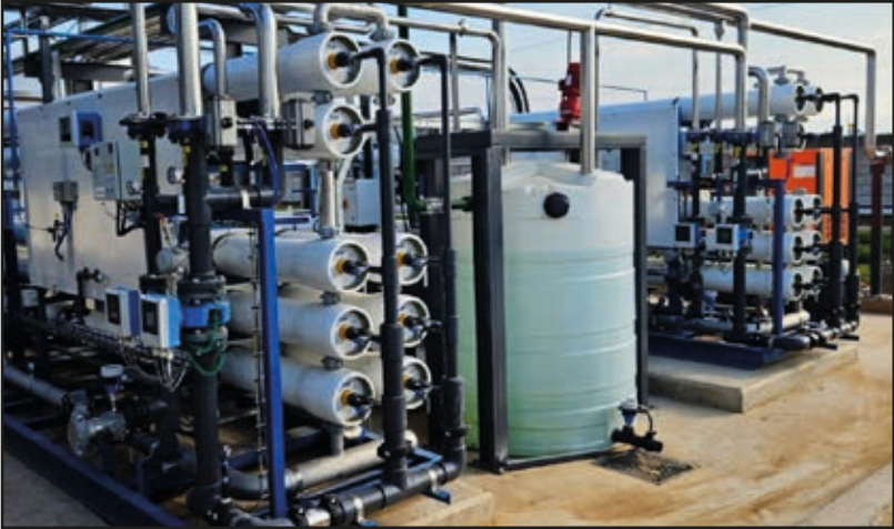
The on-site treatment plant recovers at least 70% of the 1,300 kl used each day back to potable quality
