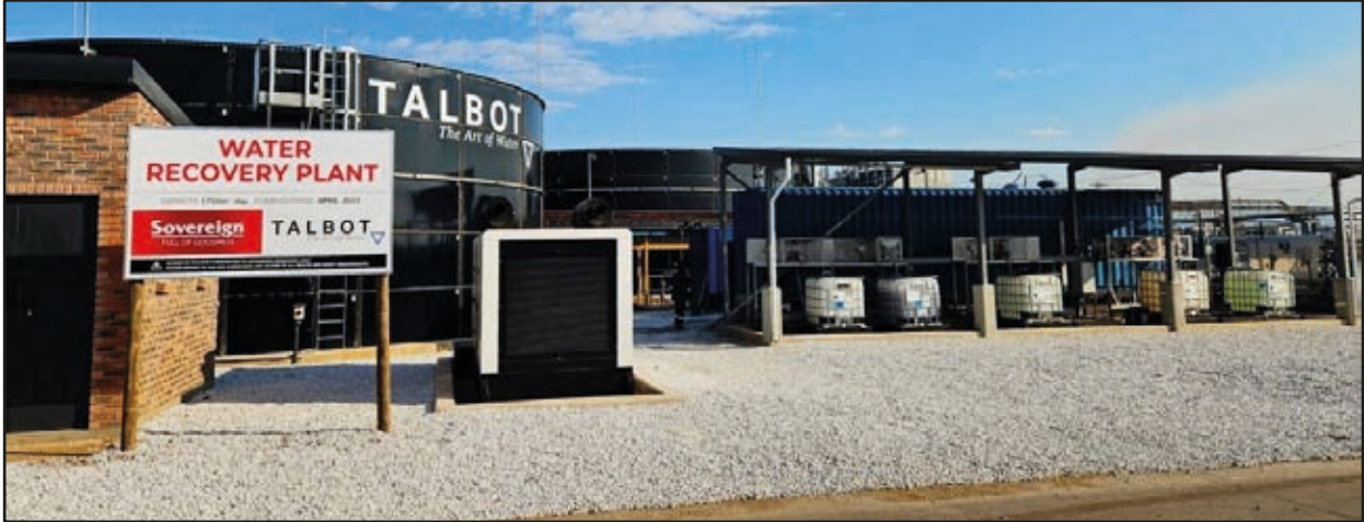
The on-site treatment plant recovers at least 70% of the 1,300 kl used each day back to potable quality
