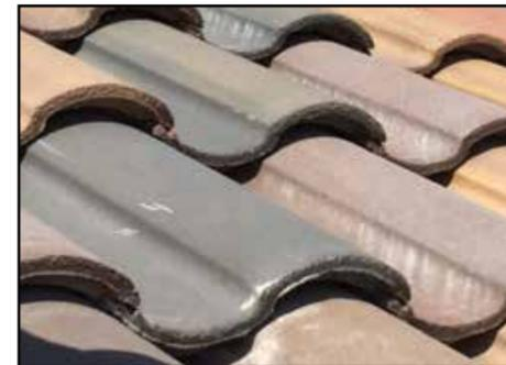
*Efflorescence is caused by soluble salts migrating through the concrete via capillary action*
